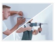
1 Use a level to mark the screw holes on the wall and drill the holes.
